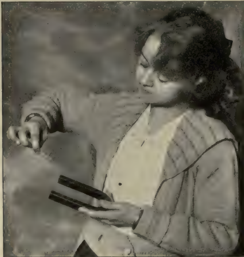
FIG. 105. Magnetizing a needle.
